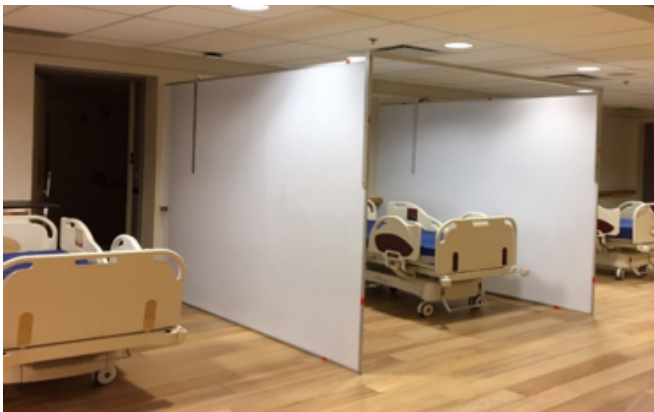
Installation of partition walls to expand ICU capacity in local hospital in Canada
