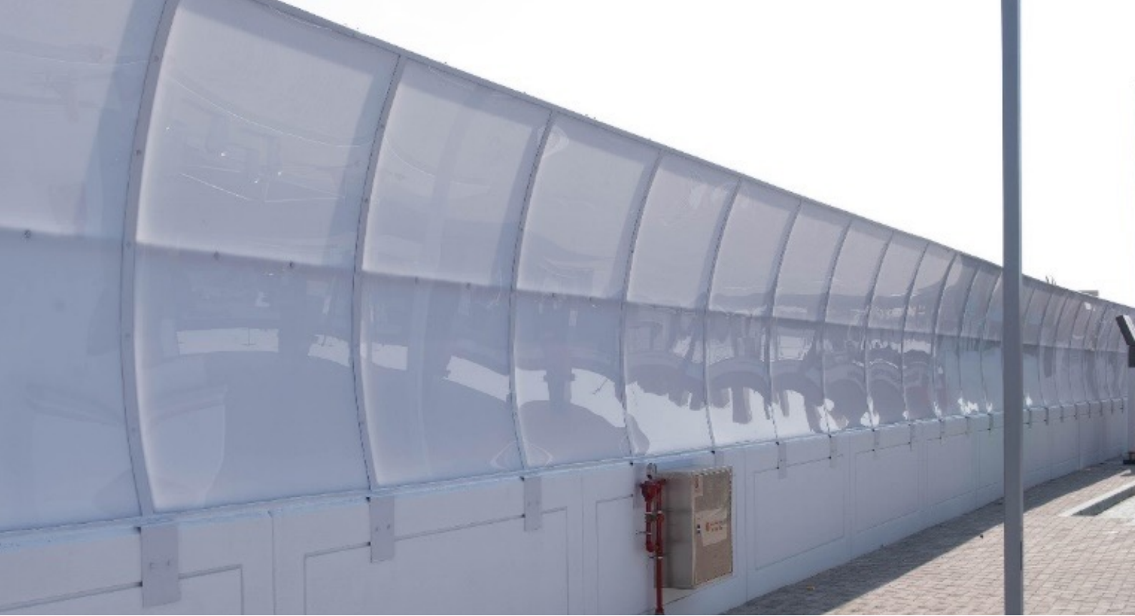
Noise Barriers, ENOC Fuel station, Dubai, UAE – With LEXAN™ EXELL™ D Opal white sheet
